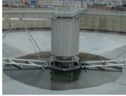
The first chain scraper system was installed at Mussalo waste water treatment plant in 2003 replacing a bridge scraper. Based on this positive experience it was decided to use chain scrapers by Finnchain in the Mussalo expansion and renovation project.
